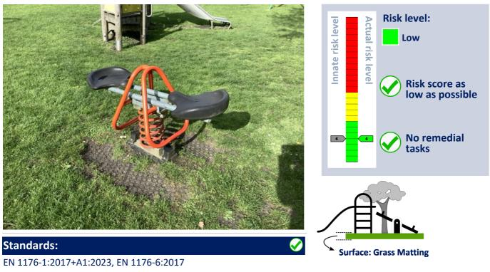
EN 1176-1:2017+A1:2023, EN 1176-6:2017 The item and its surfacing (where applicable) meet with the requirements of the relevant standards.
